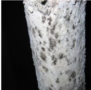
ACM- Pipe insulation (T.S.I)
