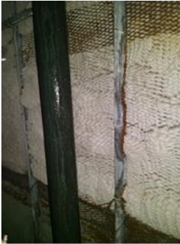
Missing insulation on cold water riser
